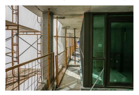
Down on the lower floors, window installers have reached the fifth floor. As they enclose the building, workers continue to insulate, and install studs, electrical and plumbing rough-ins inside the suites.
